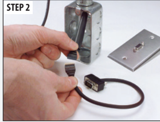
STEP 2 Slip shrinkable tubing onto cable, mate the breakaway connector matching alignment arrows and secure.
