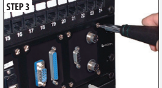
STEP 3 Using a Phillips or Flat screwdriver, install your sub-panels in the master rack panel.
