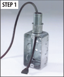
STEP 1 Feed socket end through conduit (3/4" min. dia.) into destination outlet.
